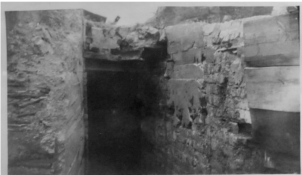
1922: the concrete German dug out along the road from Beerst towards Dixmude.
