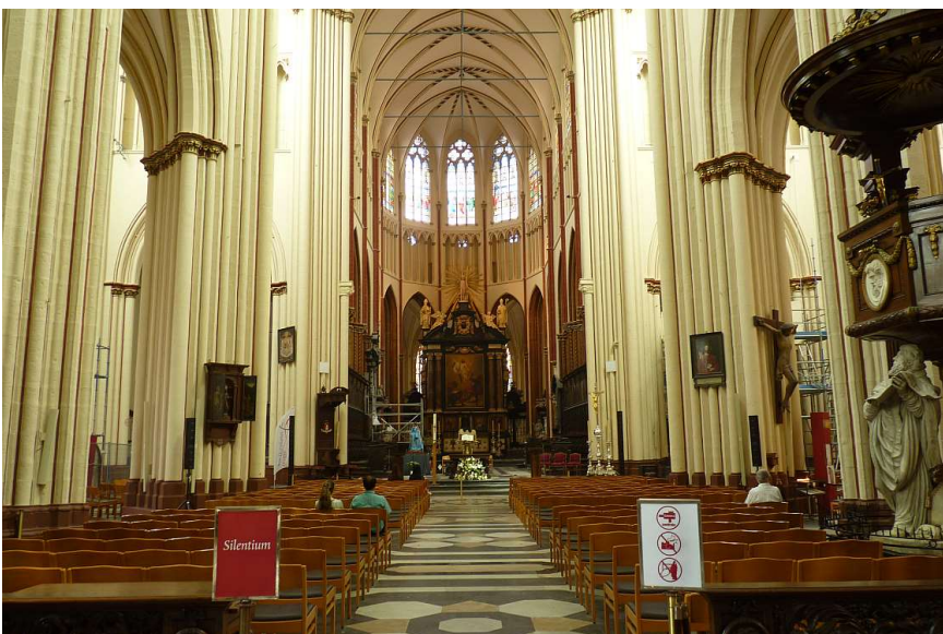
2017: interior of the cathedral today. In 1935, the baroque rood-loft with organ standing between the choir and the nave was removed and placed in the back of the nave (against the tower base). 28
