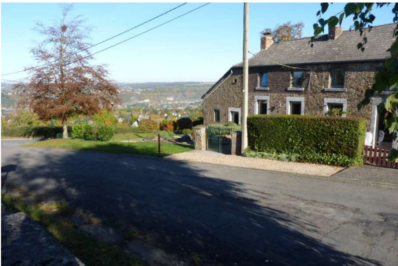
Right: the unchanged caretaker's house across the road seen from the cemetery's wall.
