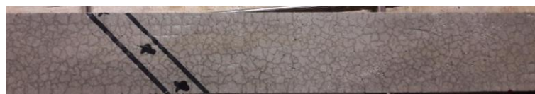
Figure 43 Appearance of shrinkage cracks after heat-rain cycles
