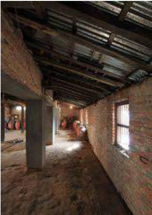
Roof structure covered with CGI sheets in the Salan guthi building in Khokana, 2016
