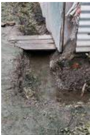
Dug gutter around shelter
