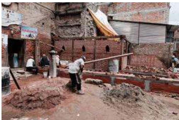
New construction of peti in front of the Rudrayanee temple, Khokana, 2016
