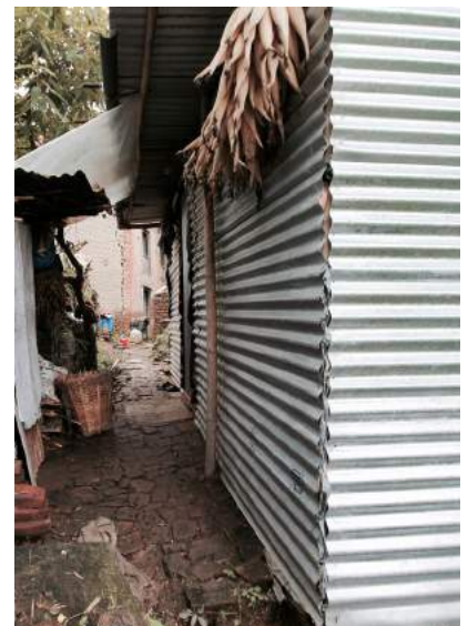
Outside of Dipu's shelter in Khokana, 2016
