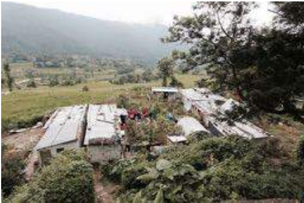
Shelters at the edge of Khokana, 2016
