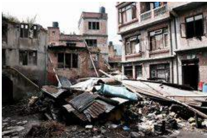
Courtyard filled with construction materials from collapsed buildings, Khokana, 2016
