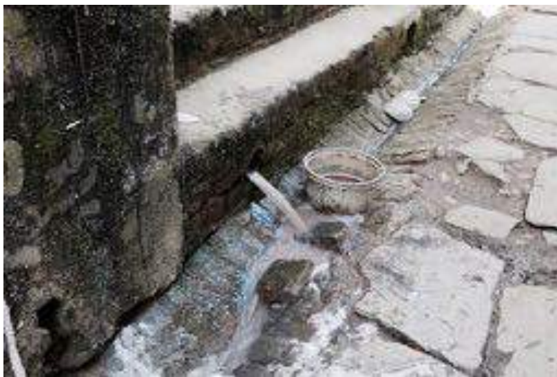
Wastewater directed to the streets, 2016
