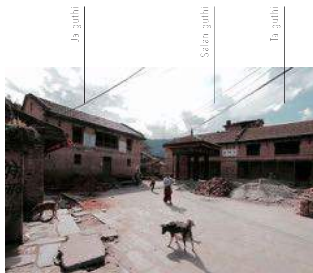
Square surrounded by the guthi buildings in Khokana
