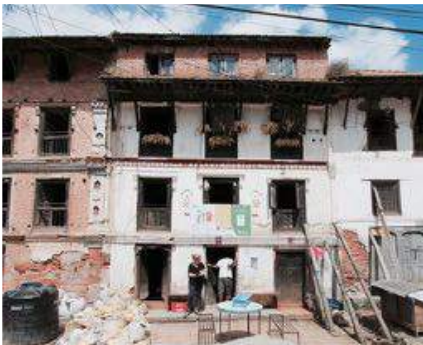
Newari house with modern extension on top on main road in Khokana, 2016
