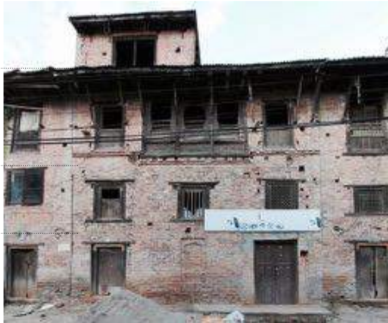
Window openings differ in each floor, 2016
