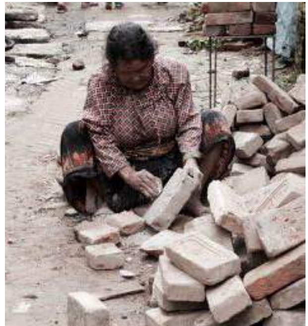
Woman cleaning bricks from demolished house for reuse in Bungamati, 2016
