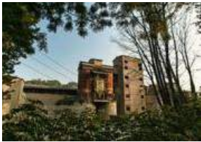
recycling in cement factory, Kathmandu. © Saliy, 2016
