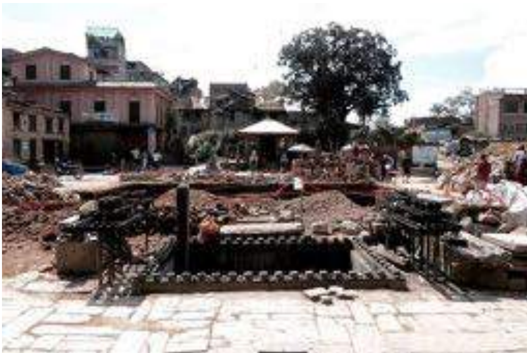
View on the main square in Bungamati where the Machhindranath temple once stood, 2016
