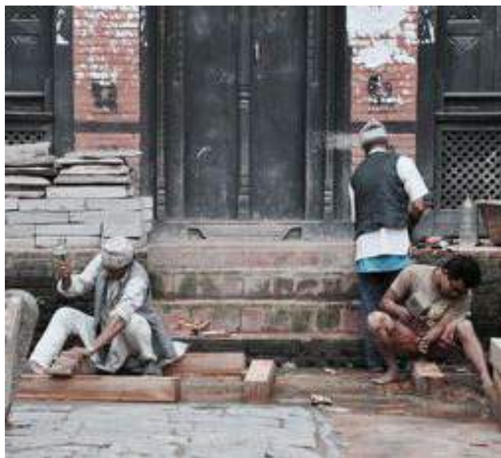
Carpenters working on reconstruction of the main temple in Khokana, 2016
