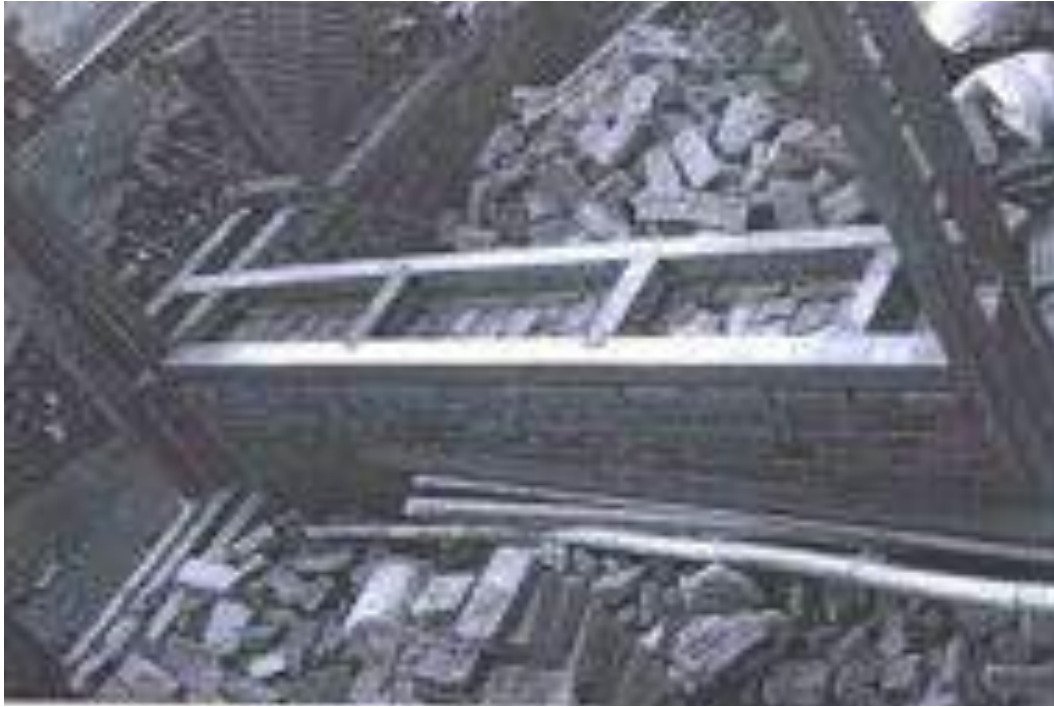
Horizontal band of the VDC building in Khokana.
