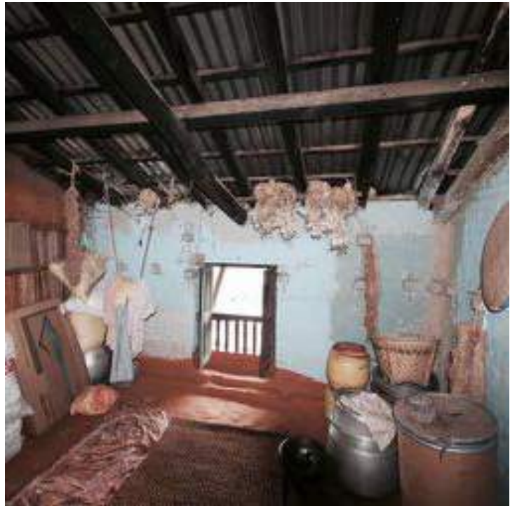
Roof structure covered with CGI sheets in a private house in Khokana, 2016
