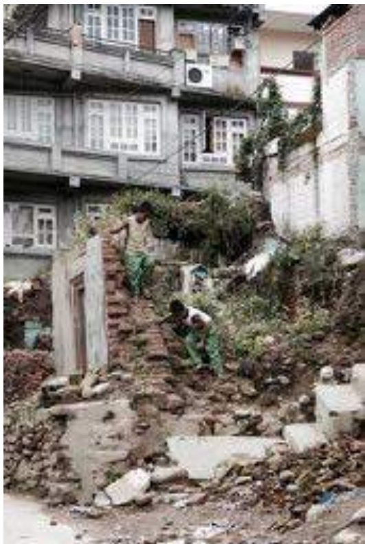
Collapsed building in Bungamati, 2016
