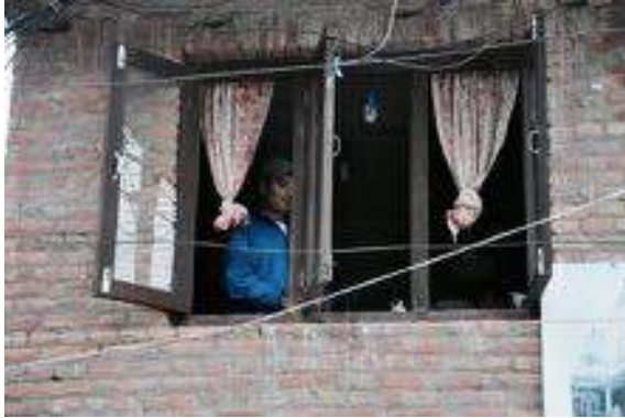
Windows on the first floor
