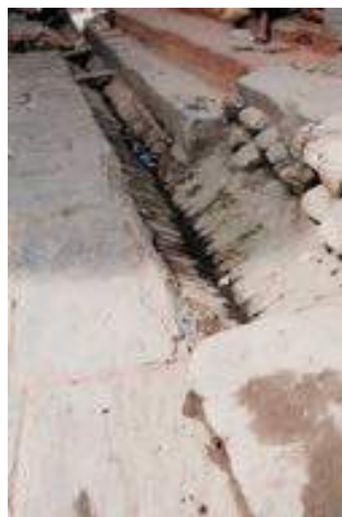
Gutter of inclined bricks
