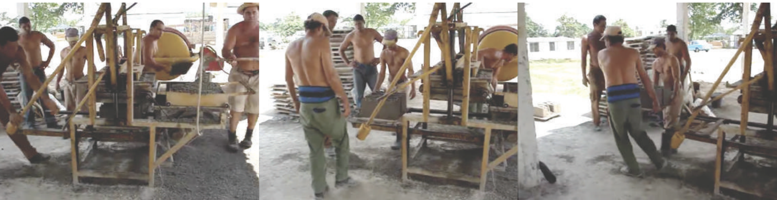
fig. 27: local construction of lime-pozzolana cement (CP-40) concrete blocks
