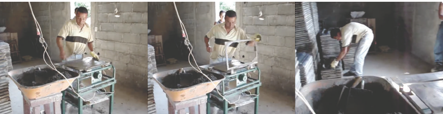
fig. 28: local construction of Micro Concrete Roofing tiles (MCR)
