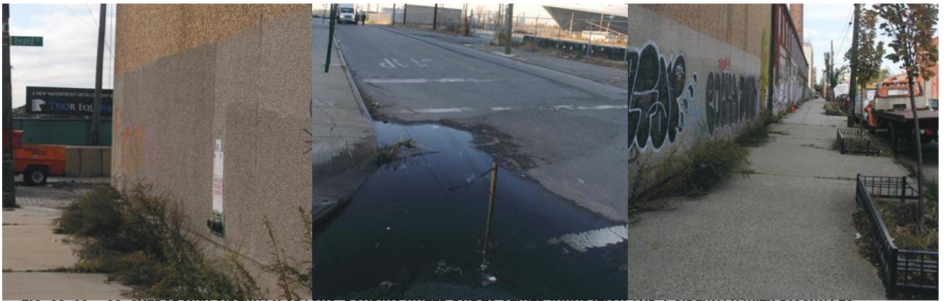
FIG. 28, 29 & 30: OVERGROWN SIDEWALK CRACKS, PONDING WATER DUE TO SEWER INUNDATION AND A SIDEWALK WITH BIOSWALES
