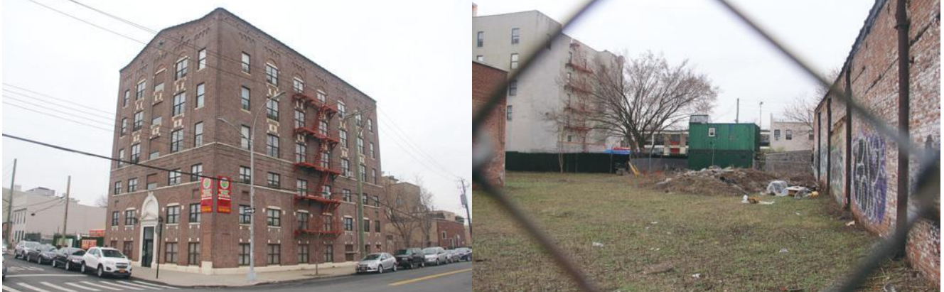
FIG. 47 : THE FORMER BETHELSHIP SEAMEN'S BRANCH OF THE YMCA; FIG. 48 : ON-SITE IMAGE WHEN ENTERING FROM KING STREET
