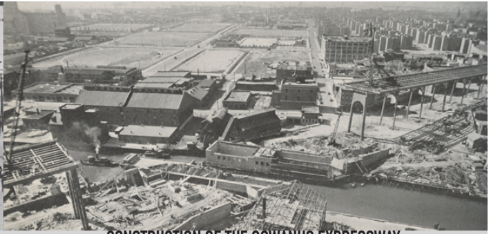
CONSTRUCTION OF THE GOWANUS EXPRESSWAY
