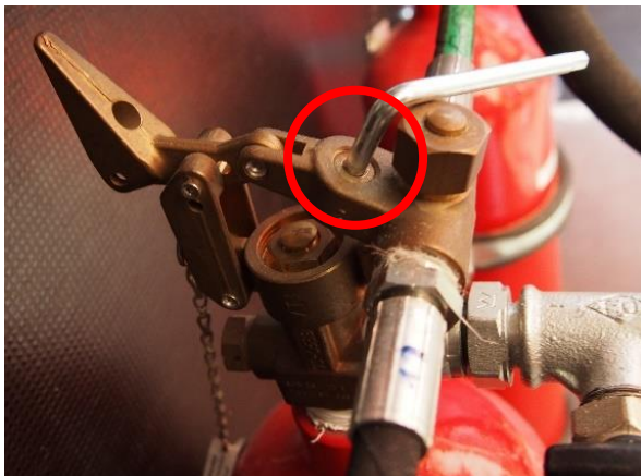
Figure 46 Adjusting the cylinder valve release screw Source: own work
