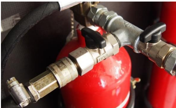
Figure 68 Connected compressor on the CO 2 cylinder filling piece Source: own work
