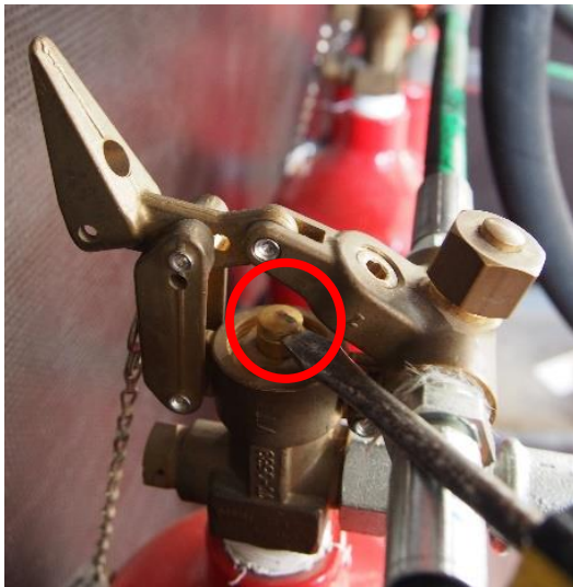
Figure 67 Opening of the pin inside the CO 2 cylinder valve Source: own work
