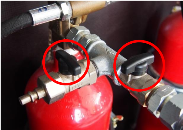
Figure 45 CO 2 cylinder filling piece, closed position Source: own work
