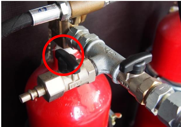
Figure 73 CO 2 cylinder filling piece, compressor coupling closed
