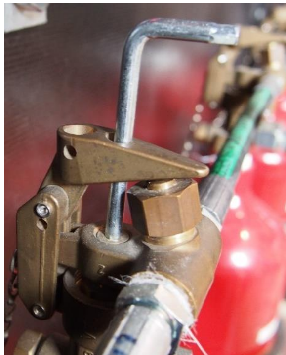
Figure 71 Adjusting the screw on the CO 2 cylinder release valve Source: own work
