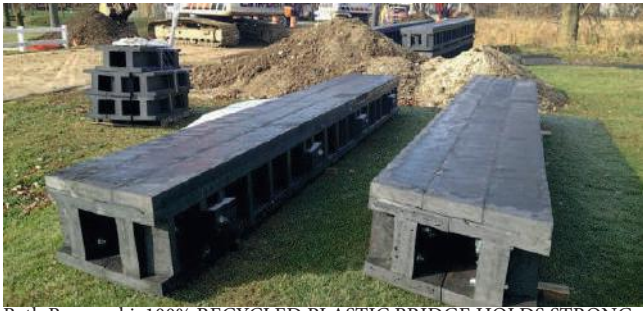
Beth Buczynski, 100% RECYCLED PLASTIC BRIDGE HOLDS STRONG IN OHIO laatst geraadpleegd 5 juni 2016 via http://earthtechling.com/2013/06/100-recycled-plastic-bridge-holds-strong-in-ohio/
