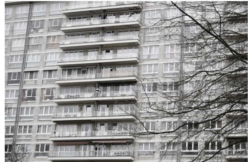
Figure 25: Brughel Parc Residence II by Etrimo (Zellik Brussels)
