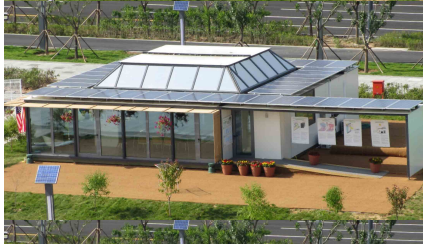
Figure 2. Solatrium in Datong
