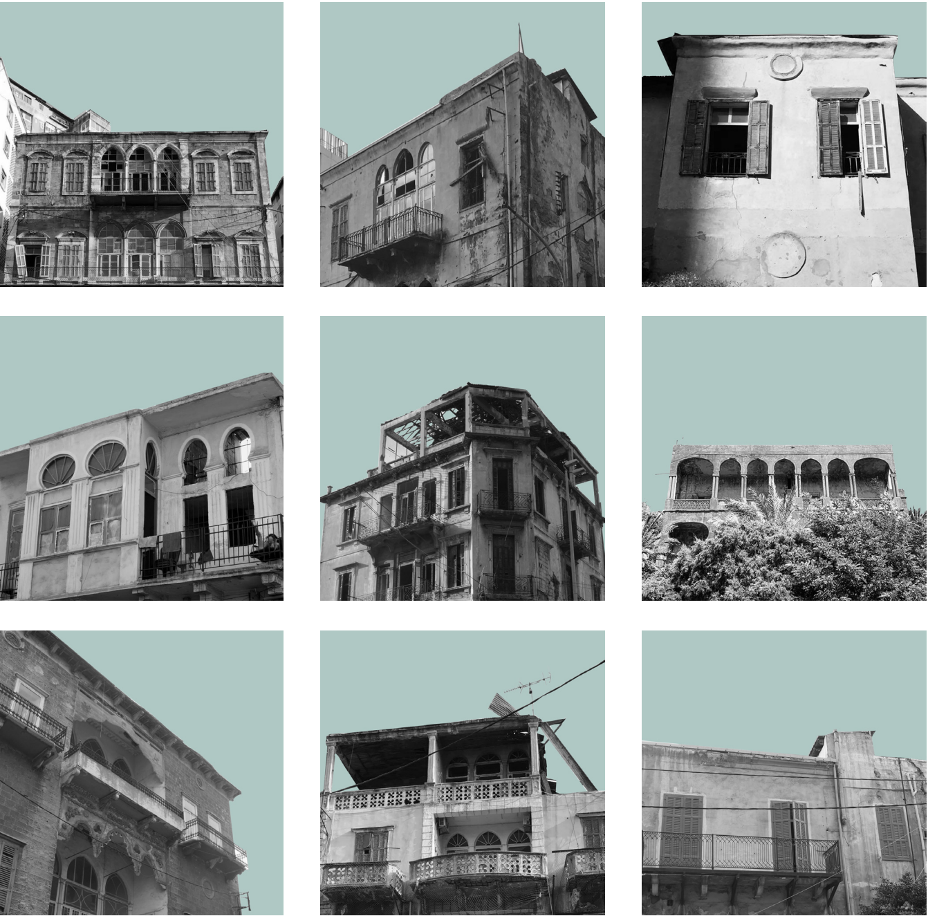
fig. 3 Some examples of unprotected traditional buildings throughout Beirut.
