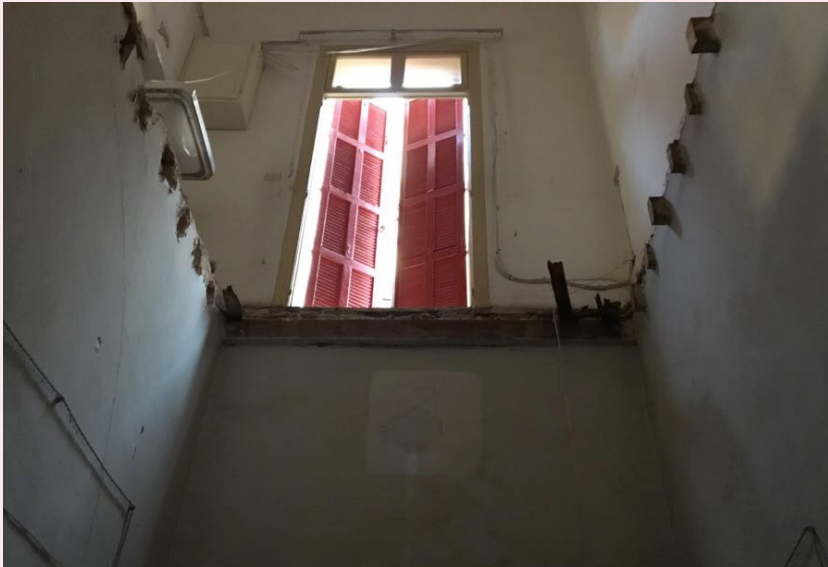
fig. 33 Photograph by Samir Rebeiz, demolished floor, 2017.
