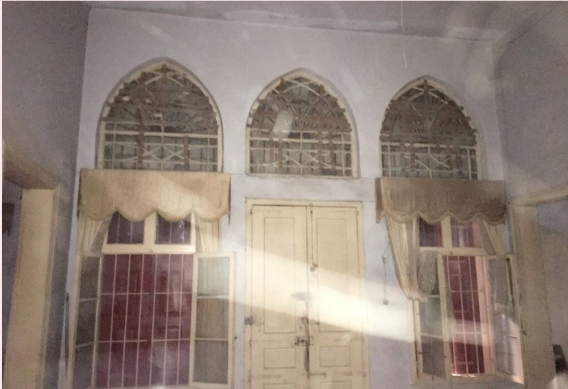
fig. 32 Photograph by Samir Rebeiz, the Red House's interior in its current state, 2017.
