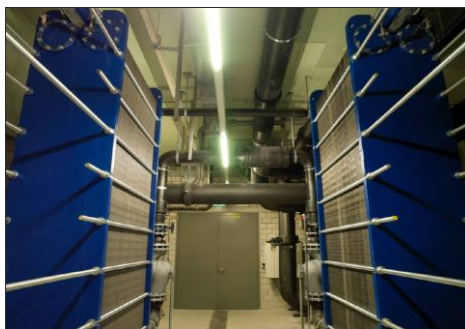
Figuur 2.7: Plate heat exchanger
