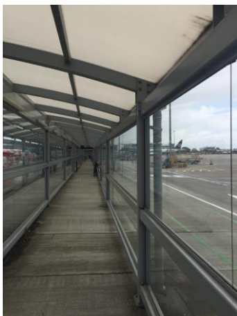
Figuur 12: Glazen tunnel
