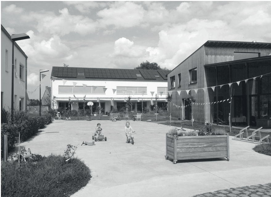
Afb. 29. Grondgebonden woningen Cohousing Vinderhoute (Cohousing Projects, z.d.).
