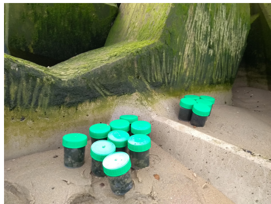
(b) Concrete blocks (Cadzand)
