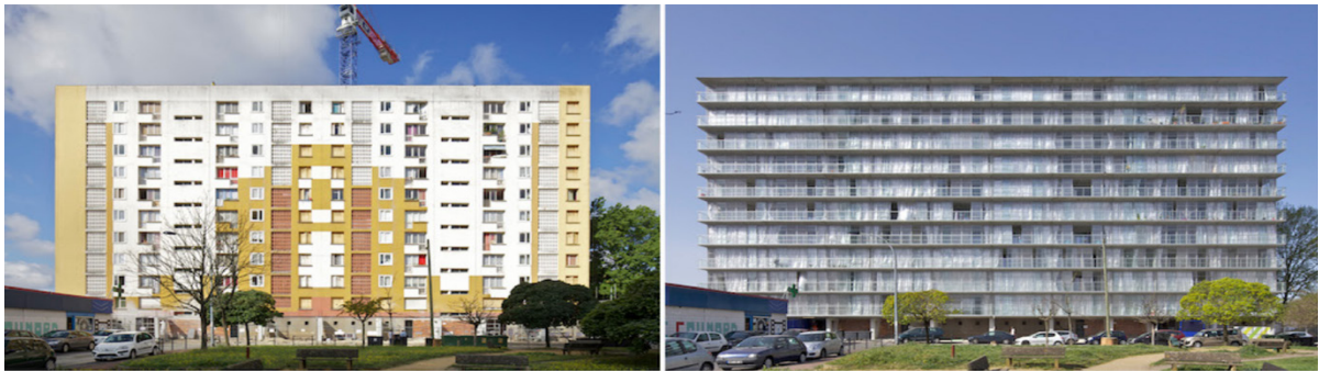
Image 2.2: renovation of grand parc, bordeaux. comparison between before (left) and after (right) renovation 7
