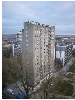
Image 1.2: post-war high-rise building before renovation 11
