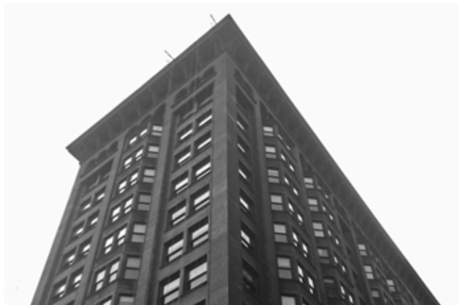
IMAGE: MONADNOCK BUILDING. CHICAGO. ILLINOIS. HANNAH VANNUT
