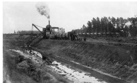
Figure 10 Old picture of the excavation of the fortress ditch.
