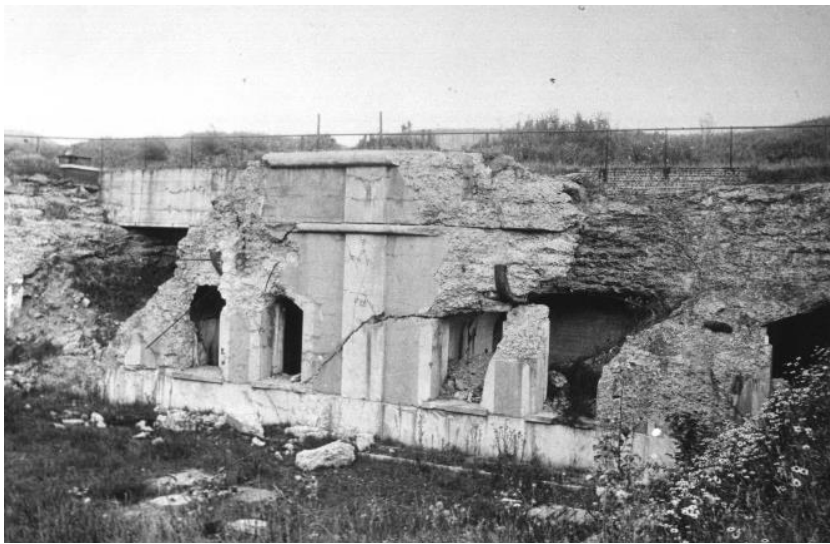
Figure 13 Old picture of the damage of the 'Big Bertha's'.
