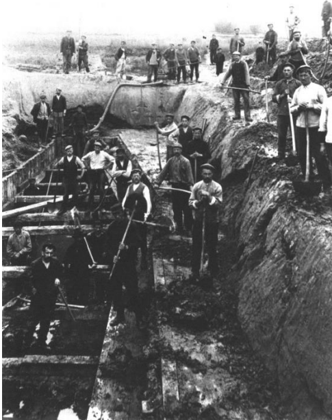
Figure 8 Old picture of the excavation of the fortress ditch.
