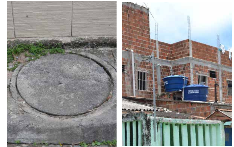
► Image 55 illustration of the utilities present in Ilha do Joaneiro, sewers and water barrels
