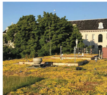
Extensive smart blue-green roof, Amsterdam © RESILIO
