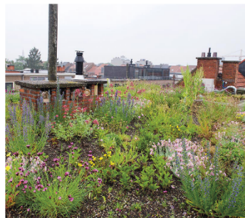
LAAD semi-intensive green roof, Heverlee © Canopy Green Roofs
