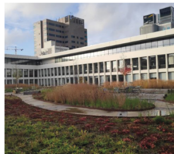
Semi-intensive smart blue-green roof, Amsterdam © RESILIO
