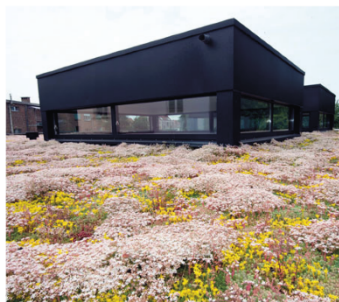
Lightweight green roof, Grimbergen © Ecoworks
