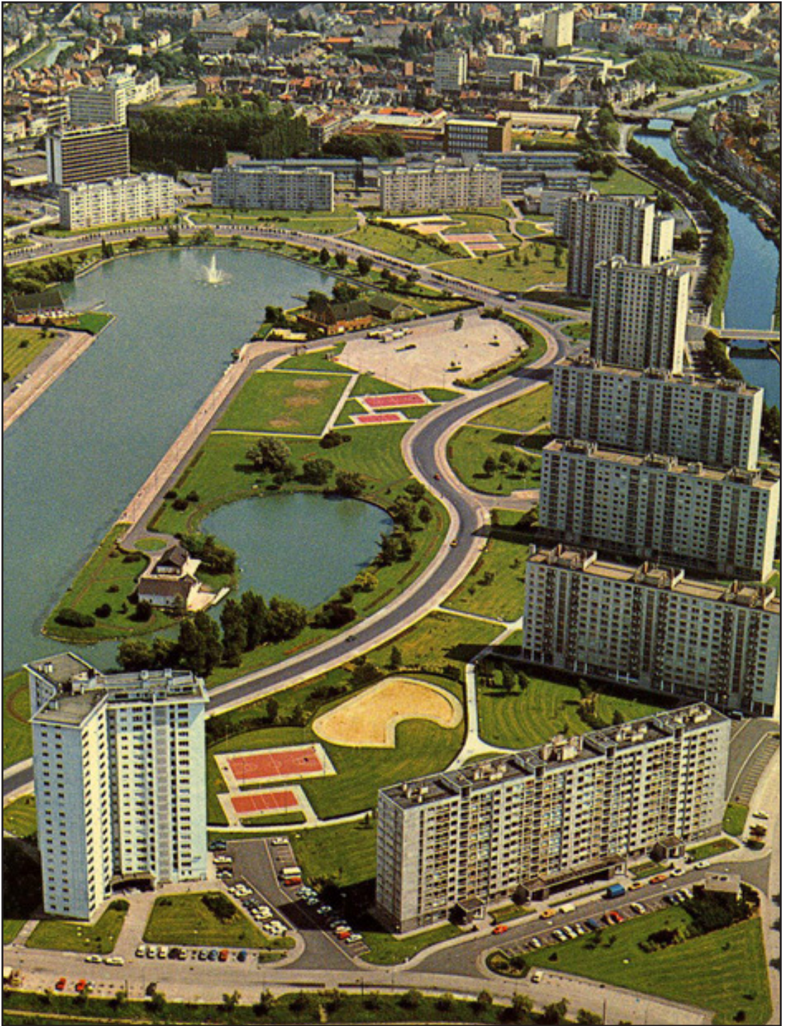
Figure IV.43: Top view of the Watersportbaan neighbourhood and its rooftops
