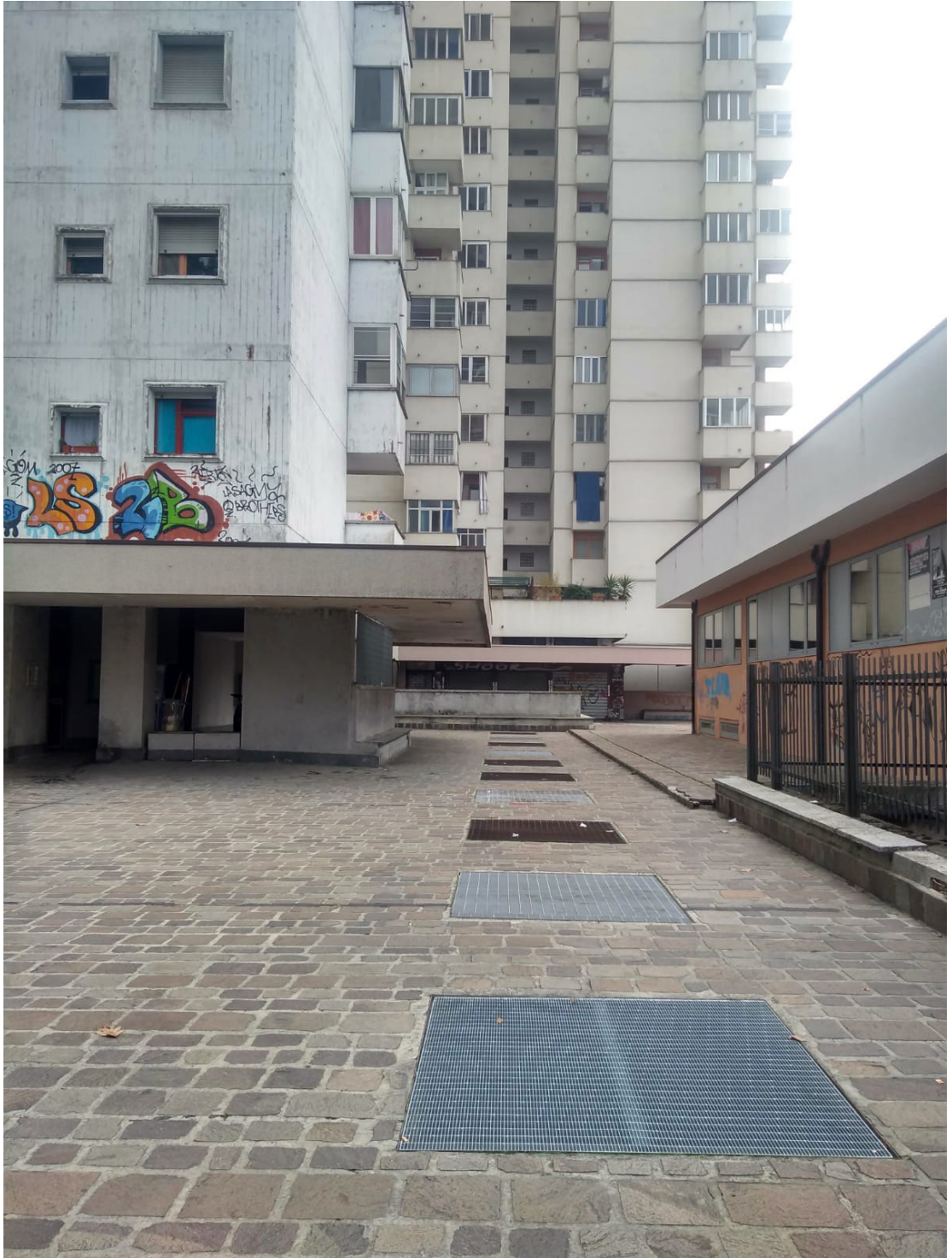
Figure IV.25: The abandoned plinths at Gratosoglio
