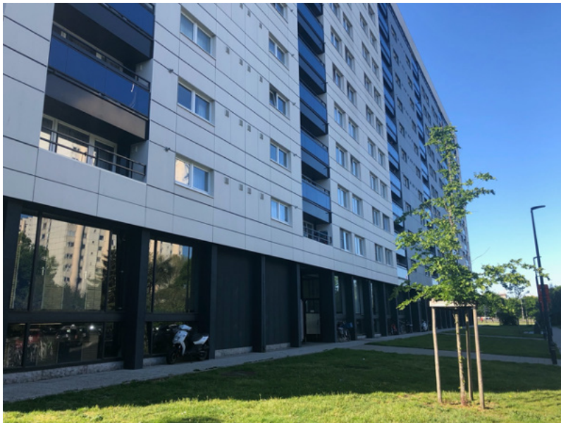
Figure III.37: The renovated facade of the Rozenhof building
