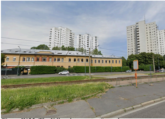
Figure IV.23: The Yellow house seen from the tram stop
