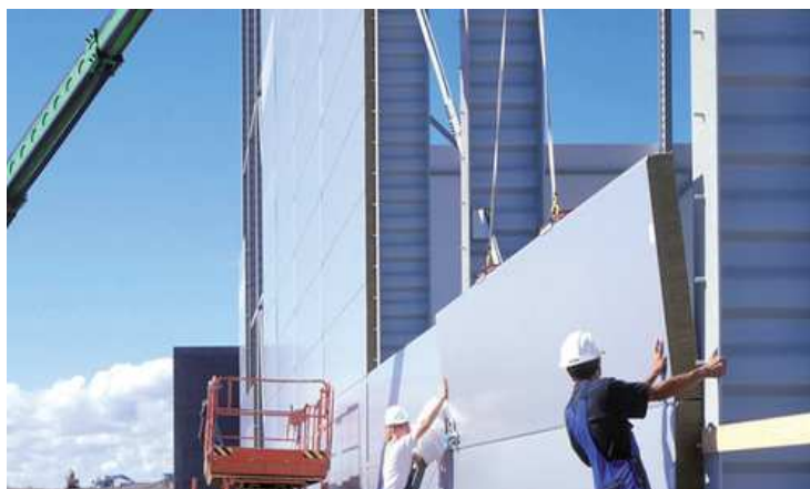
Figuur 12: Montage sandwichpaneel (Parocpanels,2021)
