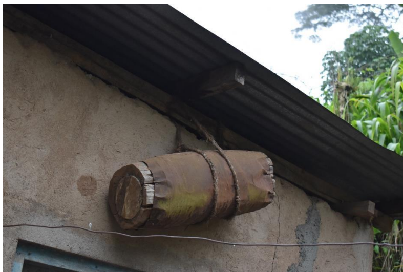
Figure 5.4: Hive which was repaired using a metal sheet
