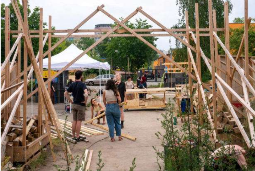
Fig. 1 The Desinc-Live Workshop on the construction site in Marzahn (Durrer, n.d.).
