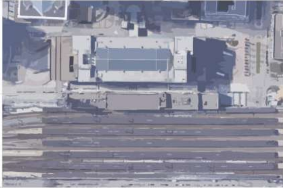
BRUSSELS NORTH RAILWAY STATION 1030
