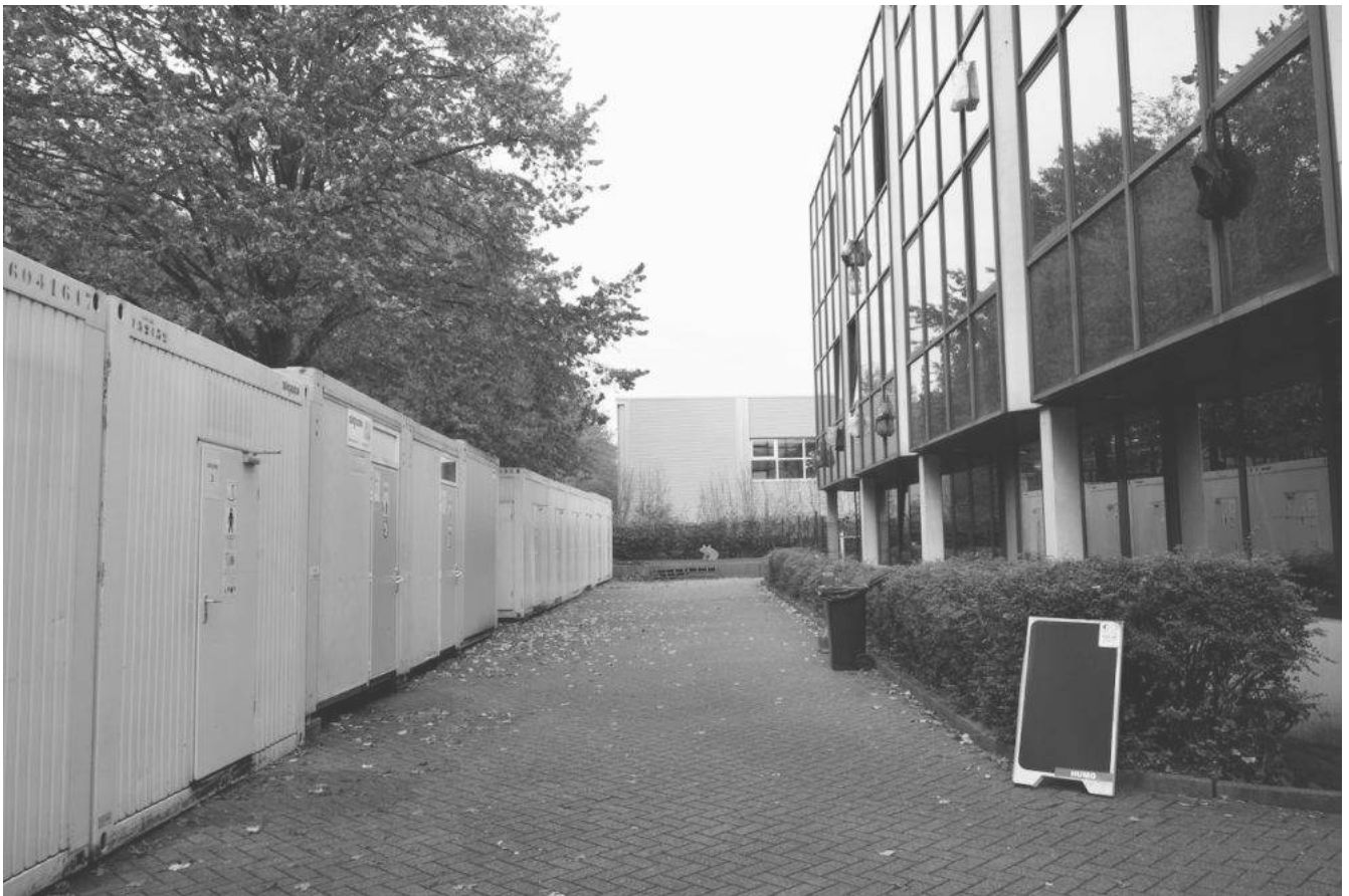
Fig. 7 Existing situation outside at the Zaventem reception centre.
