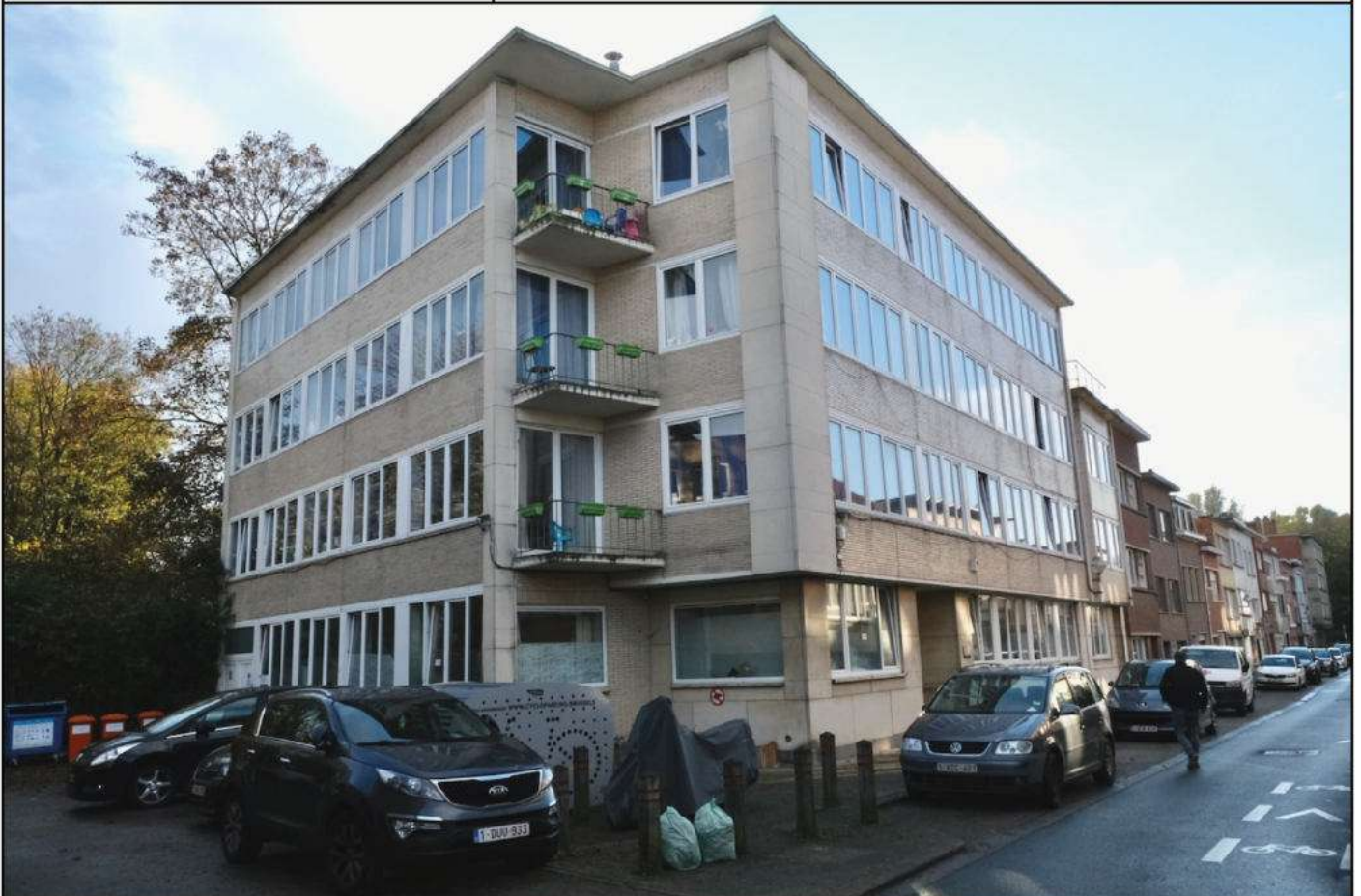
Fig. 1 The women's reception centre in Jette.
