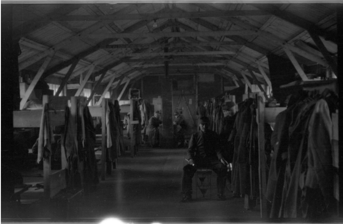
The interior of a barrack.
