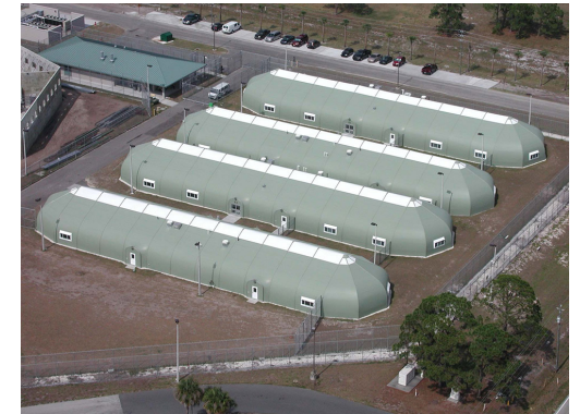
Figure 6: aerial photo of sprung structure jail - Sprung Structures, a faster way to build
