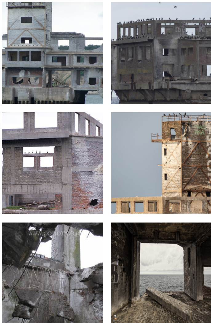
(fig.2.06) condition of the building until 2024
