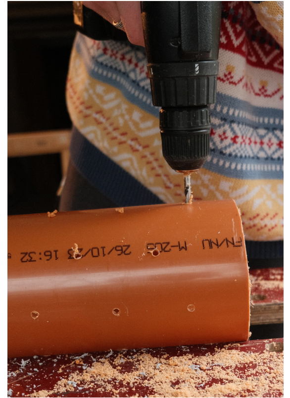
Top: Drilling of holes for ventilation in the PVC tube Bottom: Cutting PVC tubing to size, the entire tube was divided into 9 pieces of equal height
