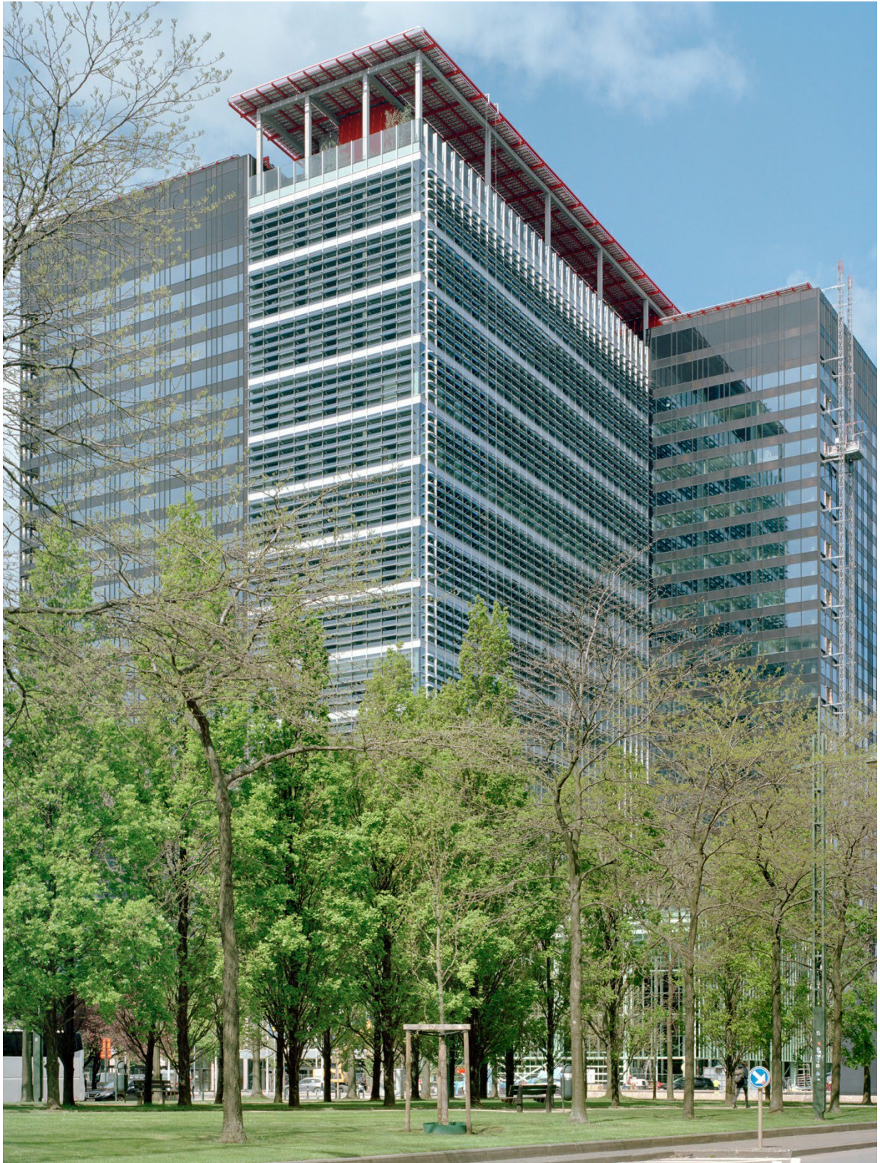
Fig. 3.10: view of the nearly finished ZIN project, redeveloping the former WTC I and II towers of the Manhattan plan, as seen from the Maximiliaan Parc, 2024. Has something truly changed? (© 51N4E)
