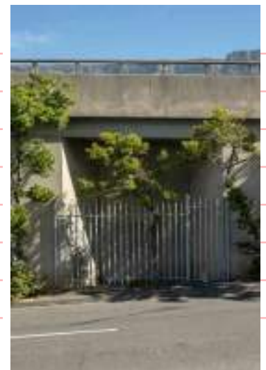
Mill Street Bridge, Right
