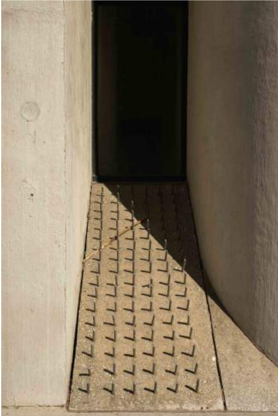
Figure 4 : Metal pins preventing one to settle, CBD
