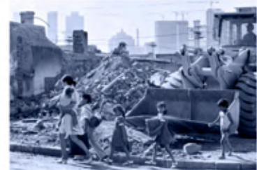
Figure 14 : Demolition of District 6
