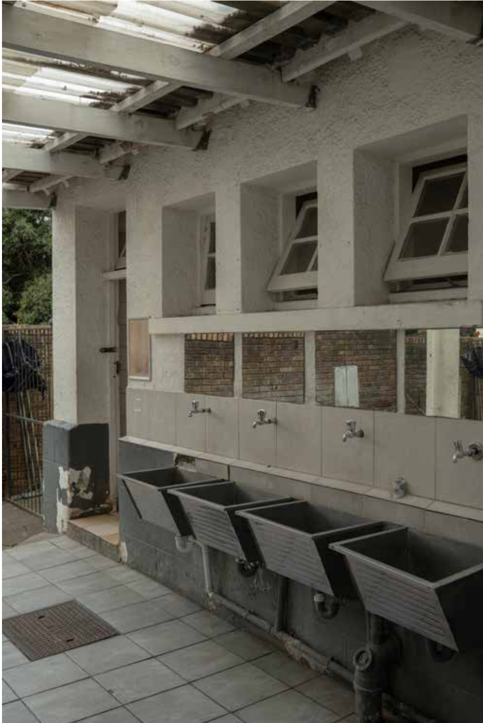
Figure 6 : Ablution facility at The Hope Exchange, CBD
