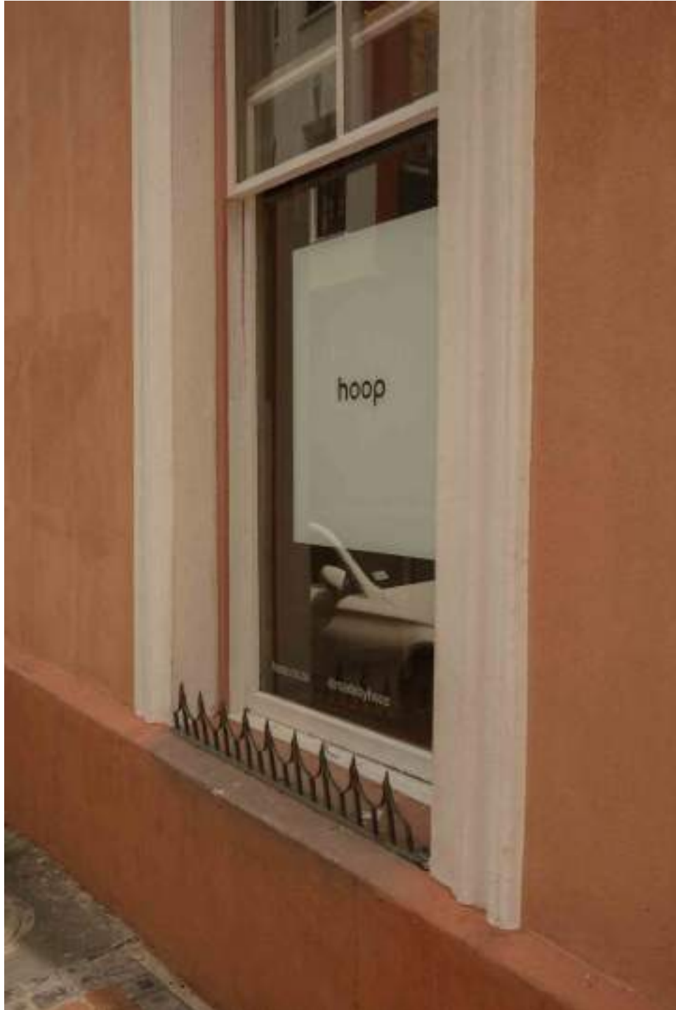
Figure 2 : Metal pins preventing one to sit on the windowsill, CBD
