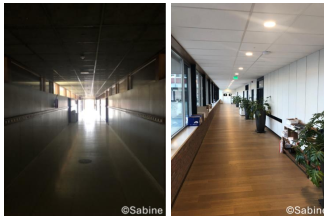
Figure 23. Corridor Sabine: bright light at the end of corridor (left), automatic lights (right)
