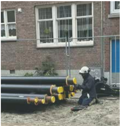
↓ Construction of the new district heat network in Bospolder-Tussendijken was well underway during our visit in March 2024.
