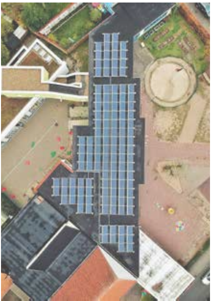
↑ The first energy community in Brussels sharing the electricity from the roof PV installation of a local school. © Bambini. (2021). via BRUZZ. https://www.bruzz.be/milieu/hoer-de-eerste-energiegemeenschap-brussel-zonnestroom-deelt-2021-02-04
