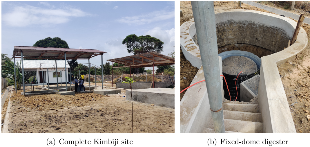
Figure 5.16: The current Kimbiji large-scale setup
