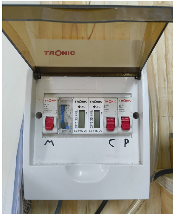
Figure 4.20: Final assembly of the electrical box
