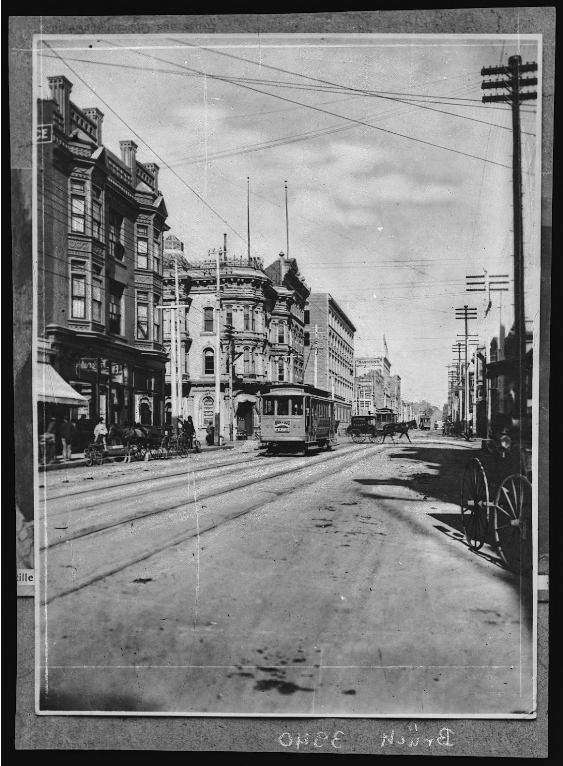
Annex 22: Original photograph Figure 19
