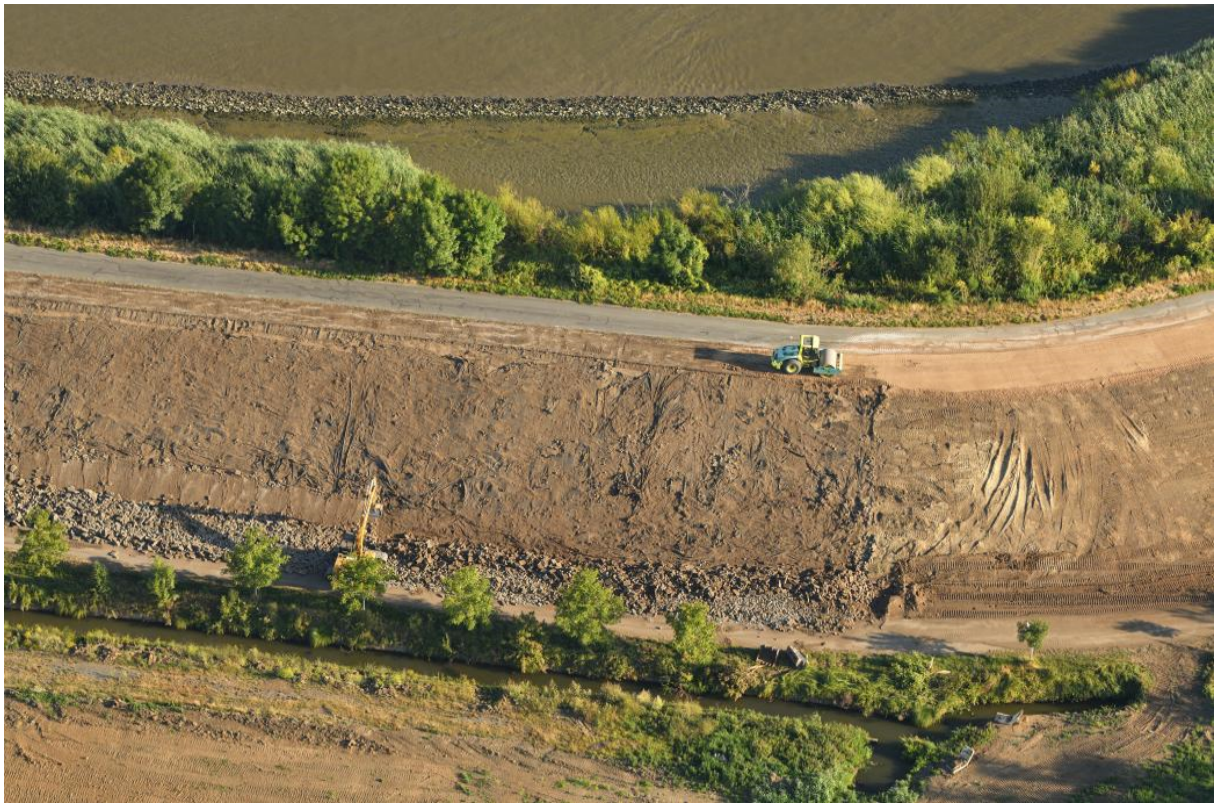
Figure 2.7: Aerial view on the new ring dike
