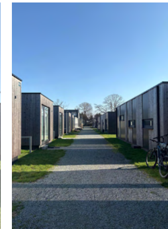
Figure 11. Emergency village, Oostakker, Phase 1.
