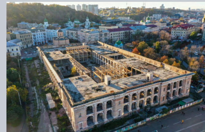
Figure 75. Aerial view of Hostynyi Dvir in downtown Kyiv, showing the deteriorated condition of the building and its position within the historical urban fabric of Podil. Note. From Kyiv activists accuse Zelensky of inaction to protect cultural heritage, by Interfax-Ukraine, 2021, Kyiv Post. Photograph by Volodymyr Petrov.
