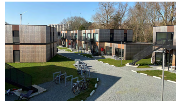
Figure 12. Emergency village, Oostakker, Phase 2.
