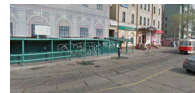
3. Exposed pavement to the street
