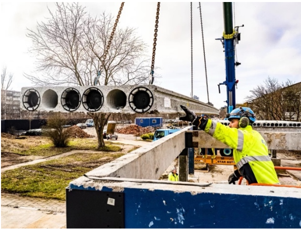
Figuur 54: Plaatsen van hol welfsel in de H22 City Expo Drottninghög. Overgenomen van Recycled concrete exhibition during H22 City Expo paves the way for circular construction , door ReCreate project, 2022.
