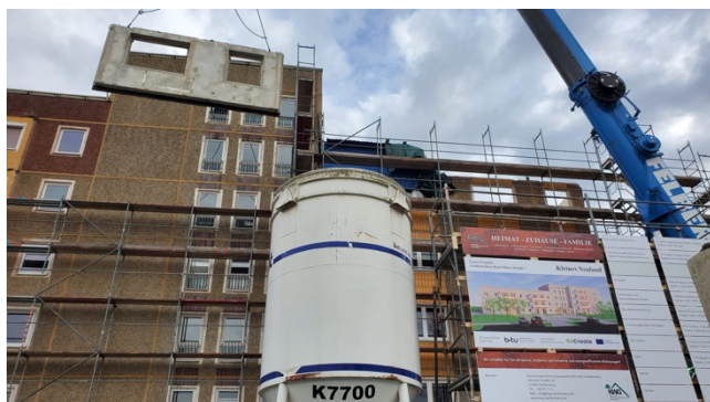
Figuur 45: Ontmanteling van appartementsgebouw in de Karl-Marx-Straße. Overgenomen van Division Selective Deconstruction - Building in Existing Contexts (ECOSOIL Ost) , door ReCreate project, 2025.
