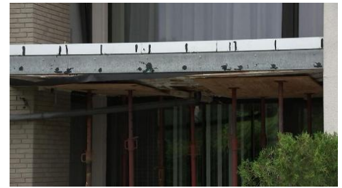
Figure 34: Decay-deteriorated balcony
