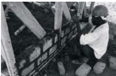
Fig. 64: Brickwork to infill the frame. Source: Shigeru Ban Architects, 2019.
