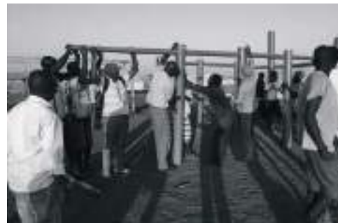
Fig. 56: Assembly of paper tube columns and beams. Source: Shigeru Ban Architects, 2019.
