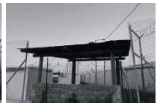
Fig. 46: The access gate of Kara Tepe 2, with ISO-box containers visible in the background. Source: Ali Muhammad, 2022.
