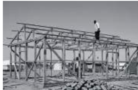
Fig. 63: Completion of timber framework. Source: Shigeru Ban Architects, 2019.
