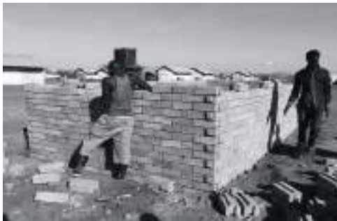
Fig. 69: Stacking of compressed earth blocks. Source: Shigeru Ban Architects, 2019.
