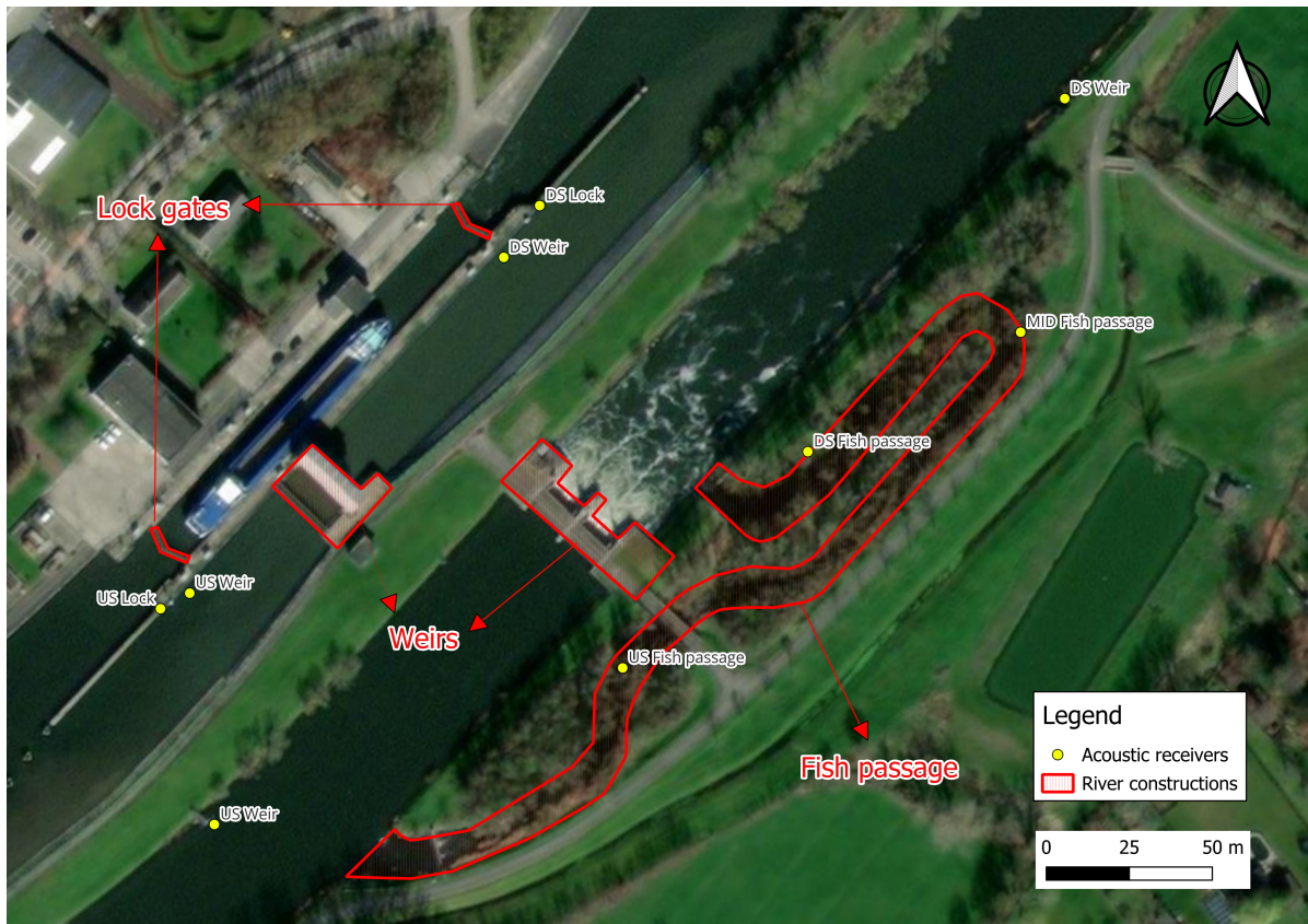
Figure 3.3: Aerial photo of shipping lock complex C in Oudenaarde, with marked river constructions and acoustic receivers. The relative position of upstream and downstream receivers is indicated in their names ('DS' for downstream, 'MID' for middle section, 'US' for upstream).
