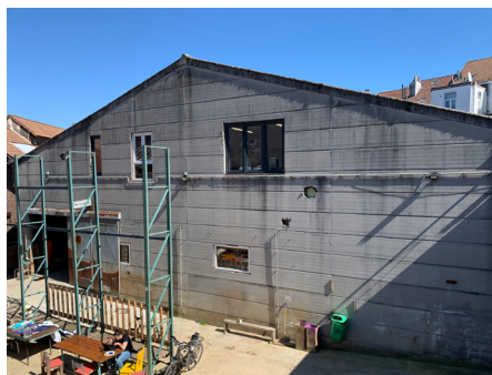
fig [5.37] Exterior of Decoatelier
