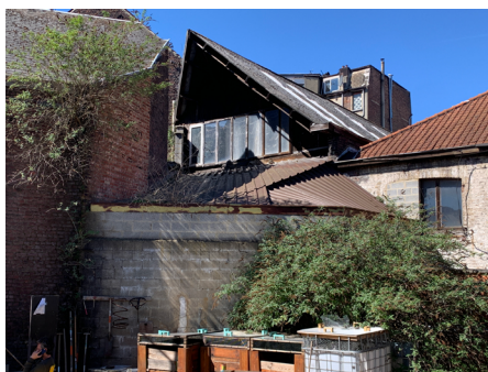
fig [5.38] Roof of Ostende 92 & Warehouse shed
