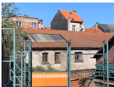
fig [5.40] Facade of warehouse Ostende 74
