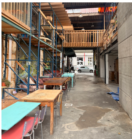
fig [5.35] Exterior of Cassonade leading to Rue de Courtrai
