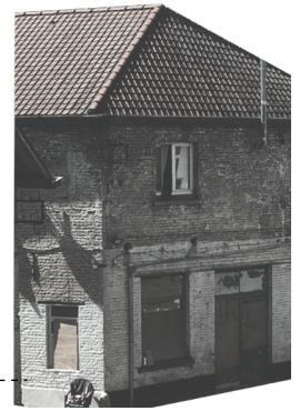
fig [5.15] warehouse Ostende 74_CACI
