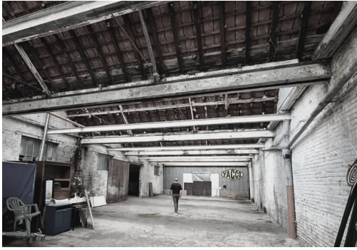
fig [5.28] interior of warehouse Ostende 74_CACI
