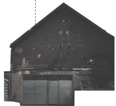
fig [5.19] warehouse Courtrai 47
