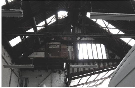
fig [5.29] interior of Ostende 92
