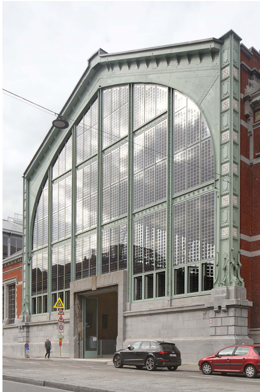
fig [4.5] Exterior of Gare Maritime_Tour & Taxis by Filip Dujardin
