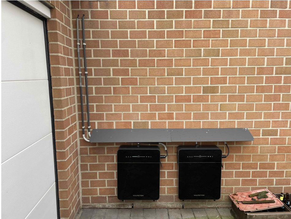
FIGURE 4.9: Physical implementation of the two Marstek E batteries installed outside the household.
