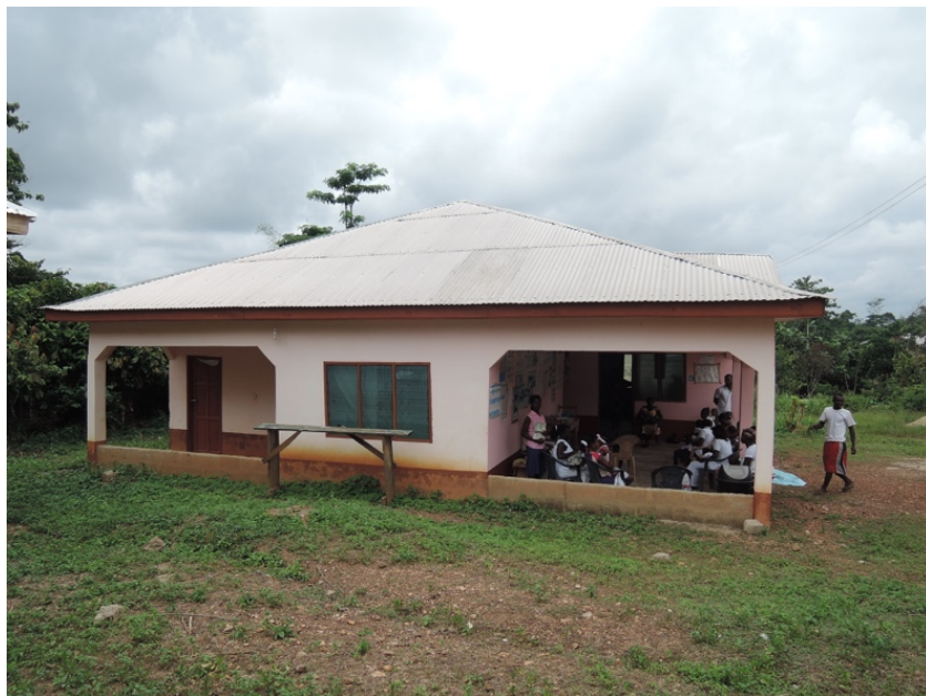
Figure 1. The CHPS compound at the edge of the village.
