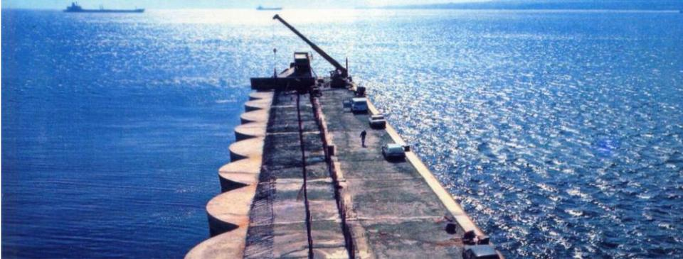
Figure 2-24: The caisson breakwater of the harbour of Naples [8]
