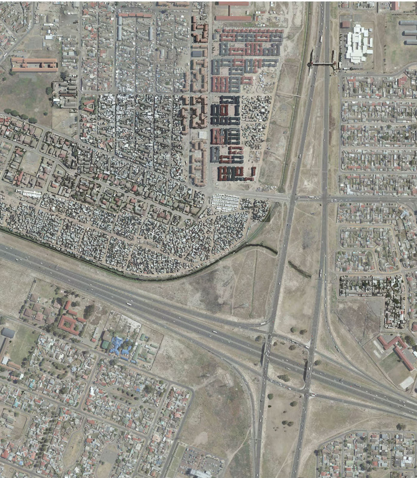
figures | urban crack
