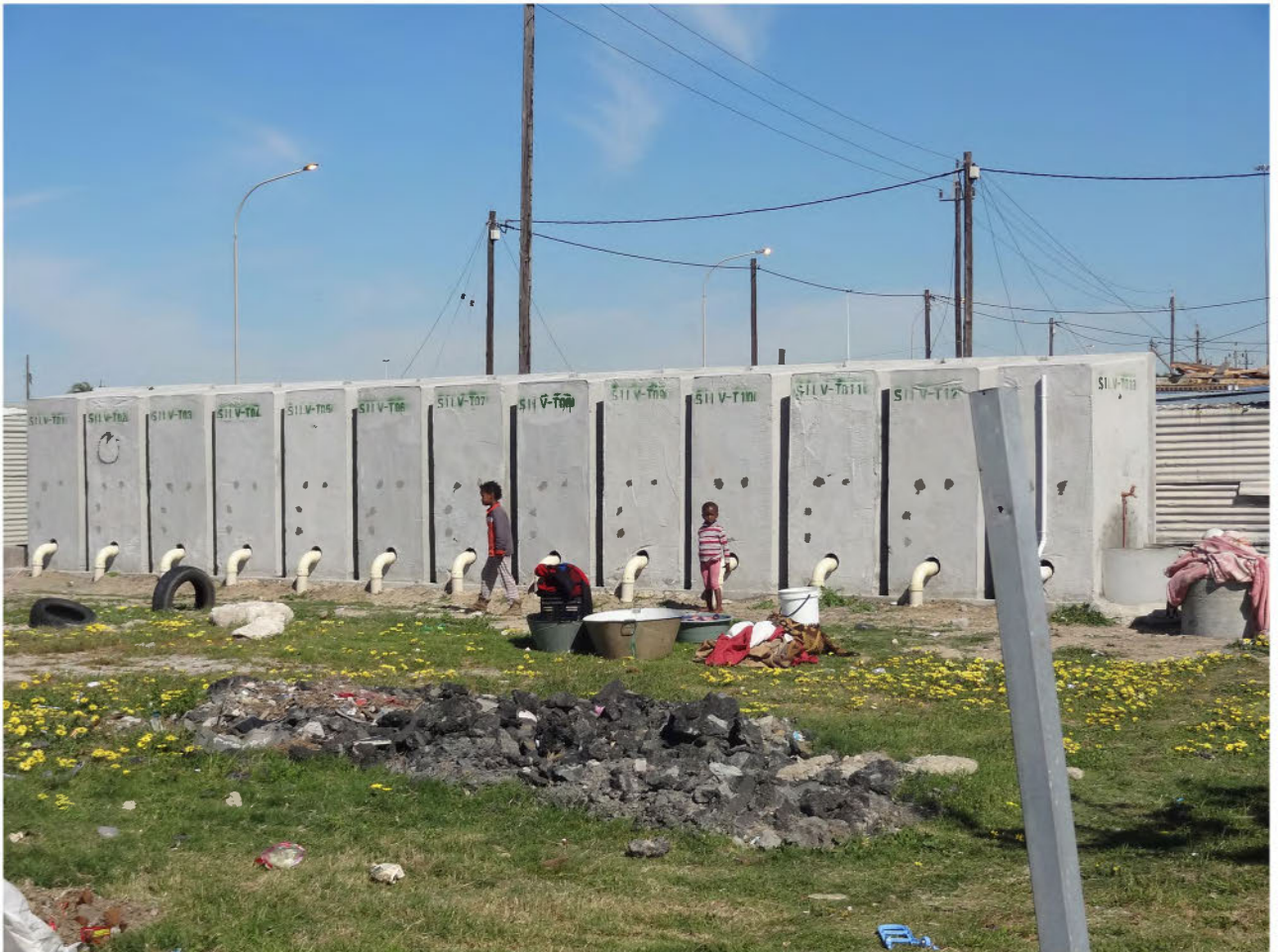
Concrete public toilets in an informal settlement in Khayelitsha
