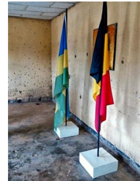
Image 54: Inside the barracks
