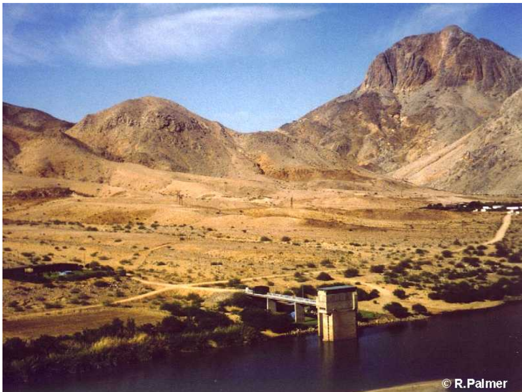
Figure 11.19: Photograph of the intake structure at Pella: R. Palmer [167].
