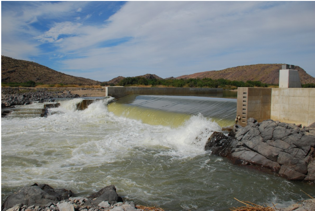
Figure 11.8: Renovated part of Zeekoebaart Weir (including a fish ladder). Photograph: field trip September 2009.
