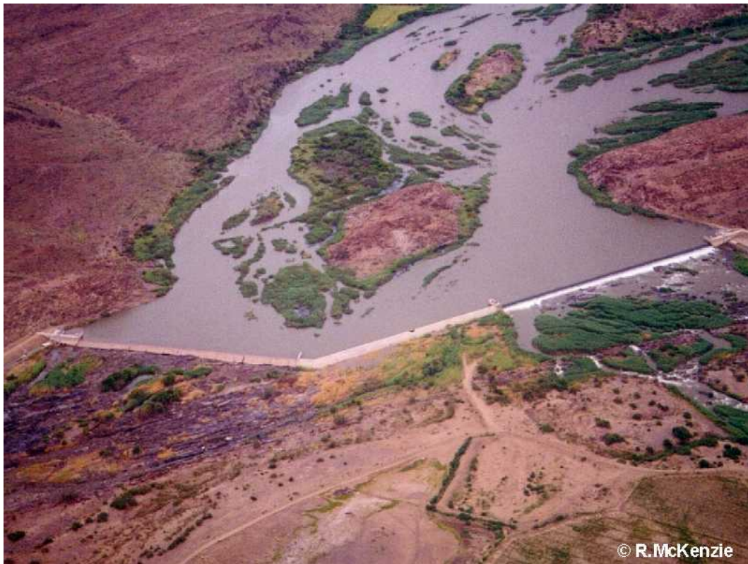
Figure 11.2: Neusberg Weir with three different notches, each with a different top level (the lowest notch is situated on the left bank of the river). Aerial photograph: R. McKenzie [167].
