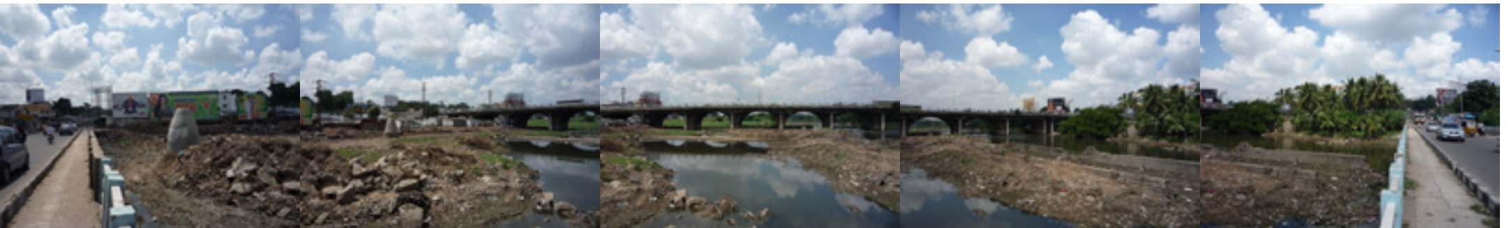
View upstream from Chaderghat Causeway
