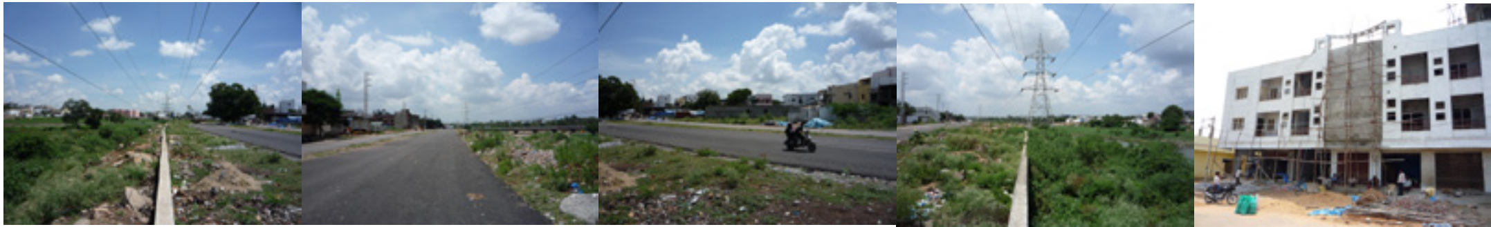
A construction site
