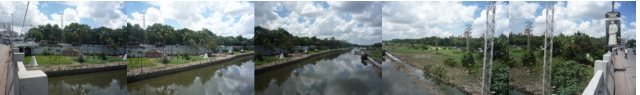
View upstream from Afzal Ganj Bridge
