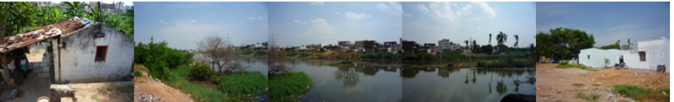
New construction in the flood zone
