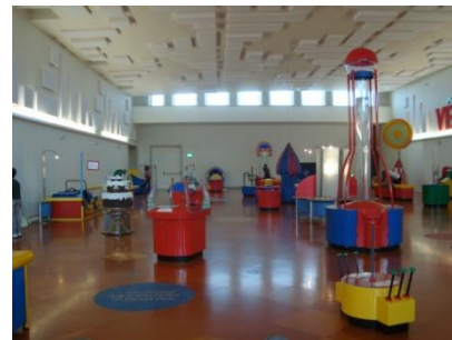
Figure 73 Acoustic Panels in 'Casa Inacabada'
