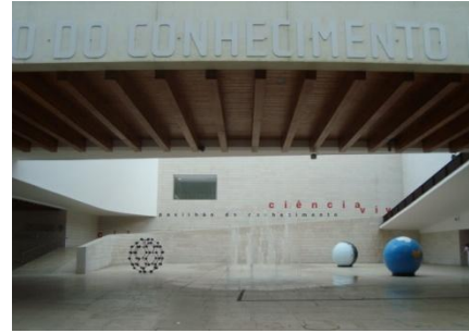
Figure 44 Concrete, Wood and Stone
