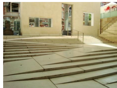
Figure 143 Steps Seen from Downstairs
