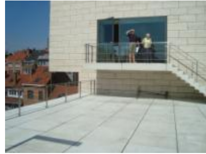
Figure 205 Entering Roof Terrace
