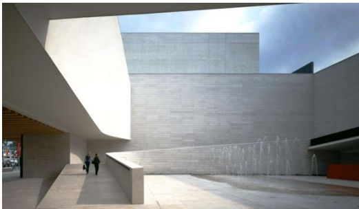
Figure 18 Front View of the Ramp
