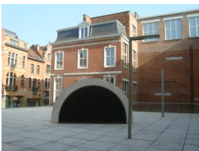
Figure 112 Attic Window Auditorium
