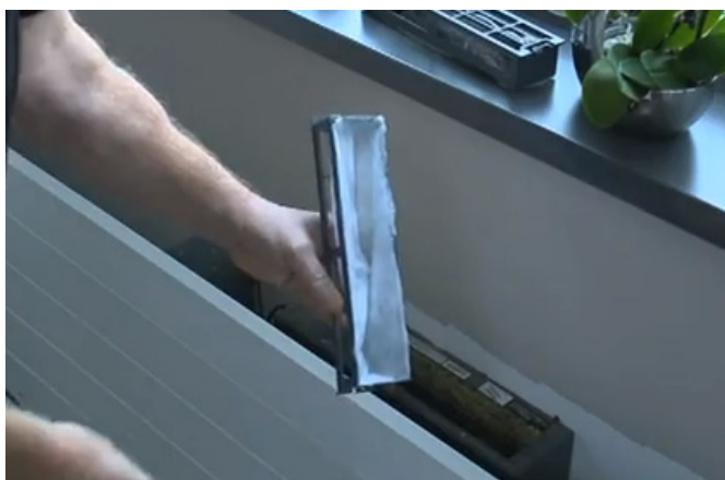
Fig. 33: Groffe filter in Oxygen-unit van Jaga
