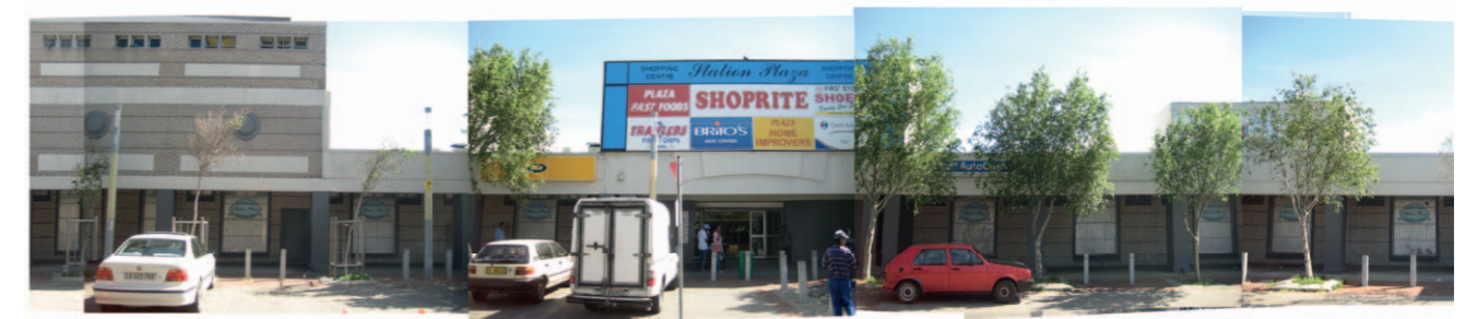
√ Station annex mall: existing building
