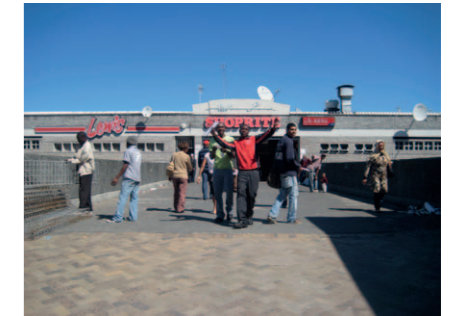
Pedestrian bridge giving access to the train station
