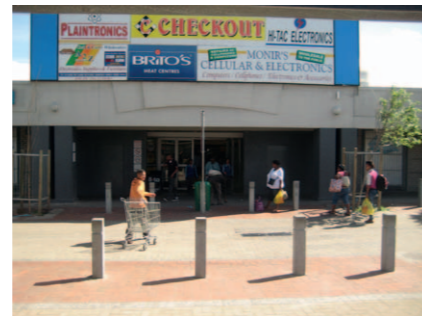
Ground floor shopping mall in train station
