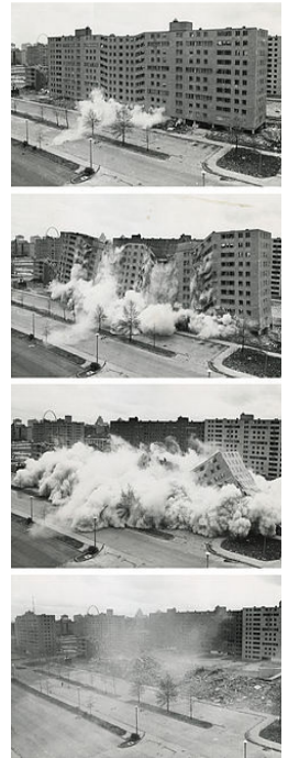
Afb 10, Pruitt Igoe Collapse Live on television, April 1972
